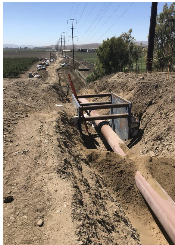
Figure 41 – L-301A Fault Crossing Pipe Replacement
