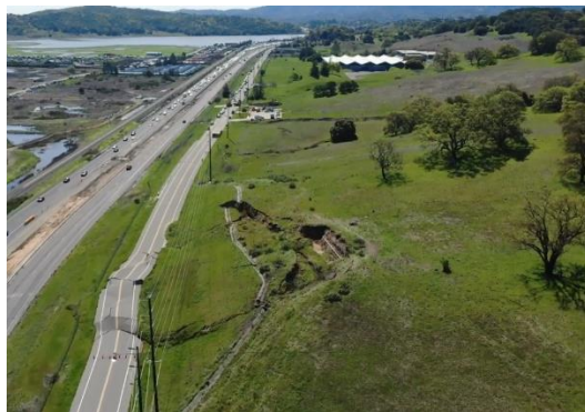
Figure 58 – Novato Landslide Affecting lines 21-G & F
