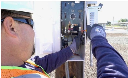
Figure 40 – PG&E Employee Installing a Cathodic Protection Rectifier
