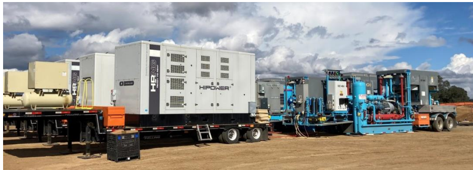
Figure 24 – Portable Cross Compression Degassing Isolated Segment of Pipeline into Adjacent Line
