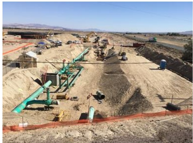
Figure 37 – Strength Test in Progress
