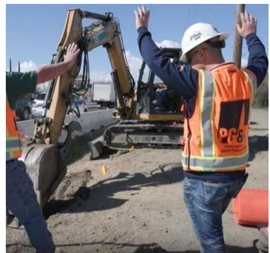
Figure 29 – Standby Crew at Work During Excavation
