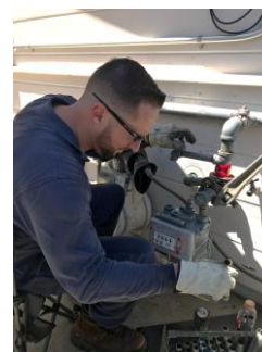
Figure 19 – PG&E Employee Working on CCE (Photo Captured Pre COVID-19)
