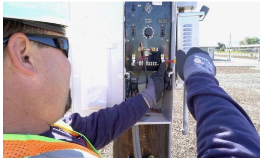
Figure 32 – PG&E Employee Installing a Cathodic Protection Rectifier (Photo Captured Pre COVID-19)
