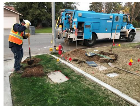
Figure 34 – PG&E’s Maintenance & Construction Crew at Work
