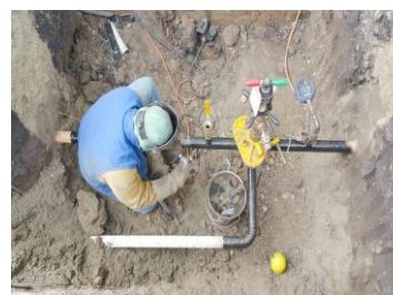
Figure 18 – Employee Working on Distribution Service
