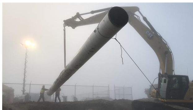
Figure 15 – Pipe SP3 ILI upgrade at Los Medanos
