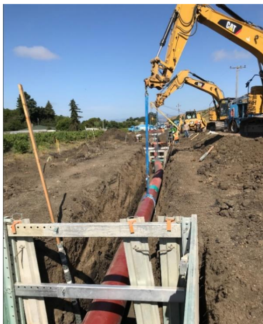
Figure 29 – Vintage Pipe Replaced in American Canyon
