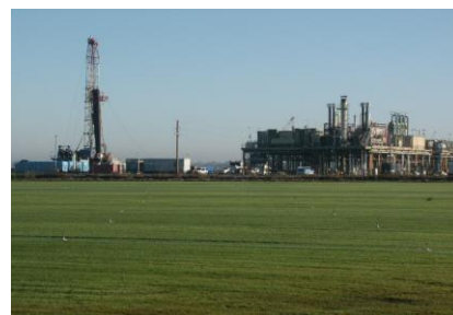
Figure 13 – Rig and Well Platform
