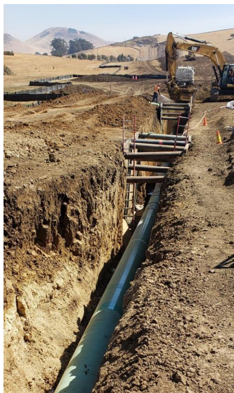
Figure 33 – 2020 Pipeline Replacement for Green Valley Fault in Fairfield
