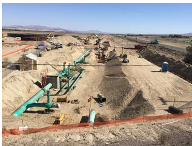
Figure 28 – Strength Test in Progress
