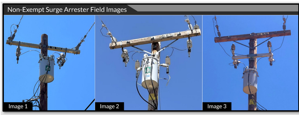
Figure 10: Example Non-Exempt Surge Arrester Field Images
