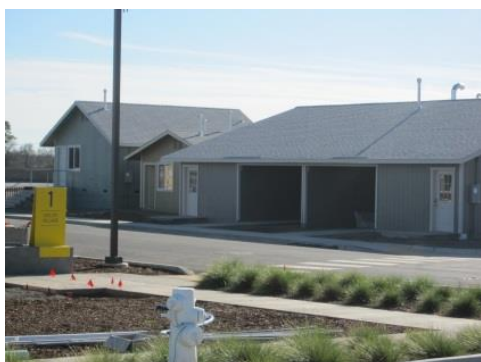
Figure 54 – A portion of PG&E’s Utility Village at the Gas Safety Academy
