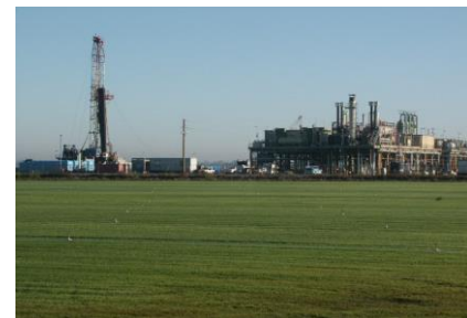
Figure 11 – Rig and Well Platform
