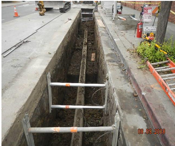
Figure 34 – Pipeline 2402-01 Replacement Crossing the Hayward Fault in Downtown Hayward in August 2018
