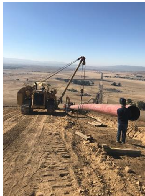
Figure 30 – Crew Replaces Vintage Pipe in Livermore
