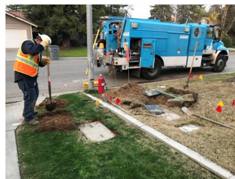
Figure 35 – PG&E’s Maintenance & Construction Crew at Work
