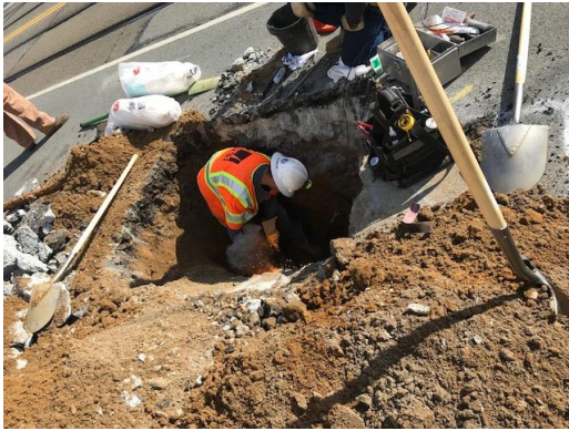
Figure 33 – PG&E Employee Installing a Galvanic Anode
