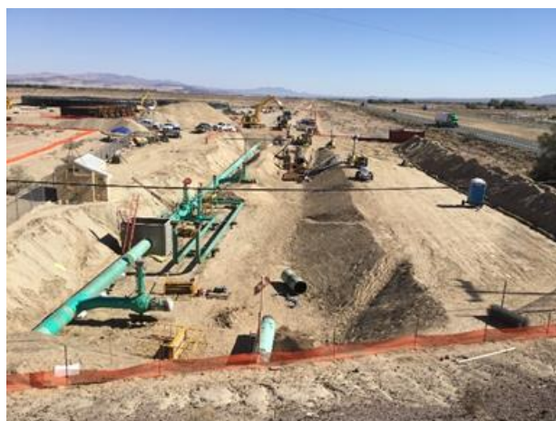
Figure 29 – Strength Test in Progress
