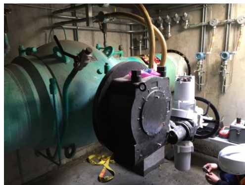
Figure 46 – A Complicated Valve Completed in 2018
