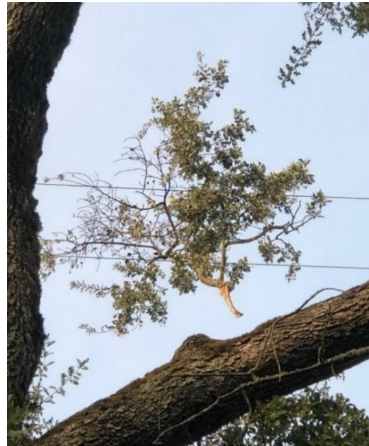
Figure 6: In Santa Rosa, Sonoma County. Tree branch on conductors
