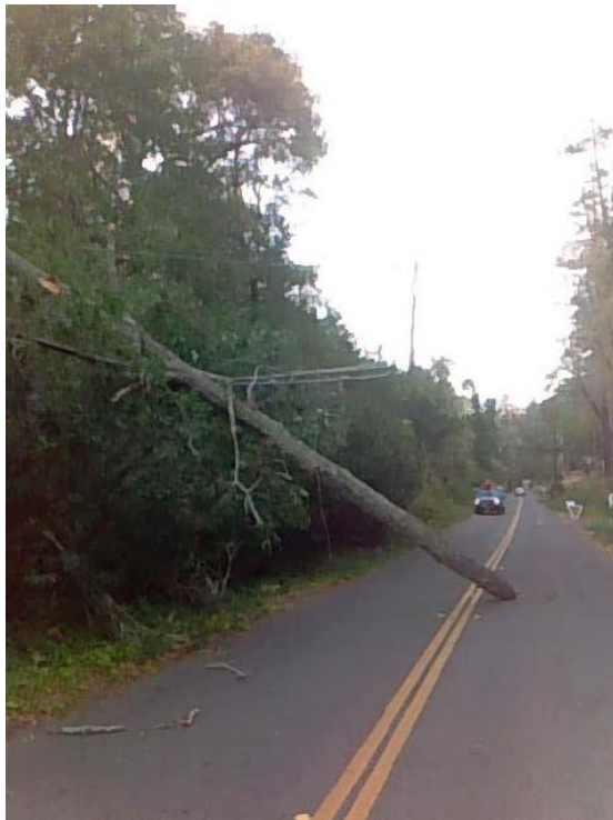
Figure 7: Tree failed and brought down conductor
