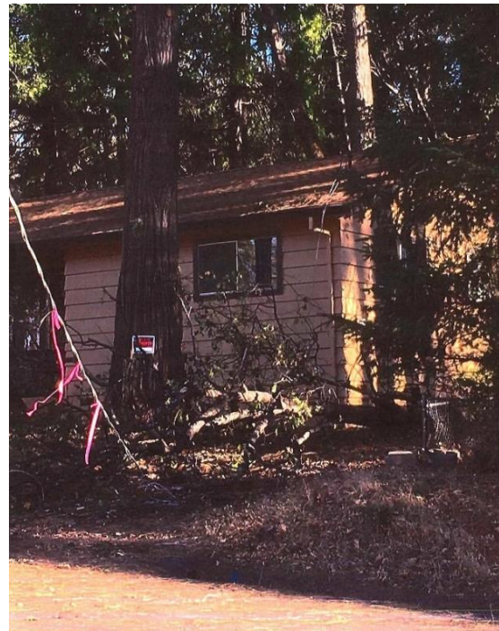
Figure 8: In Magalia, Butte County. Tree fell and brought down conductor
