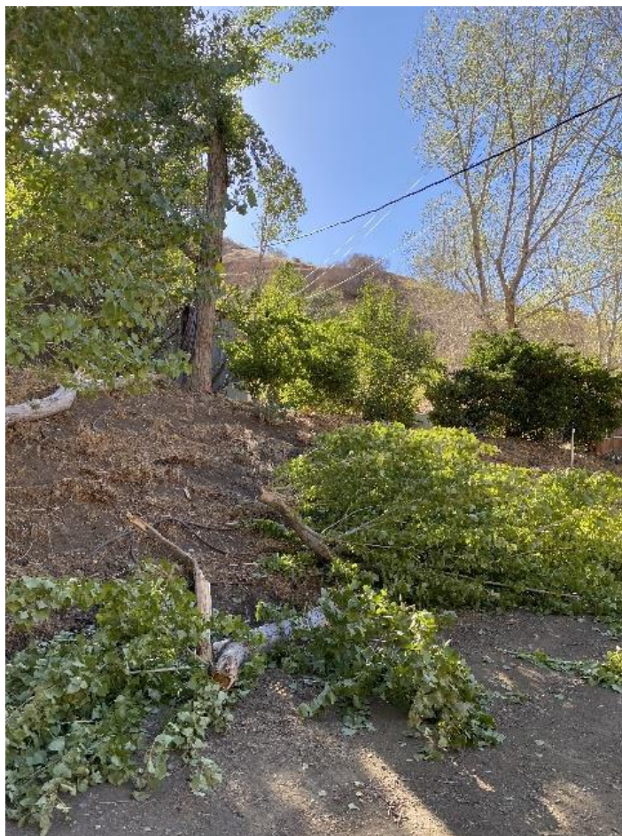
Figure 20: Vegetation-Damage in Kern County – Tree fell on Service Line
