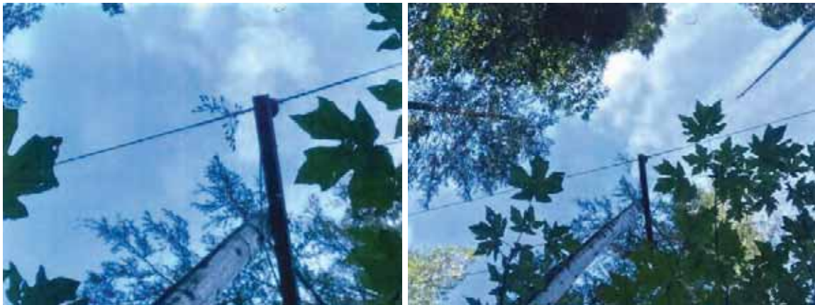
Figures 2 and 3: In Chico, Butte County, a tree branch landed on a PG&E conductor.
