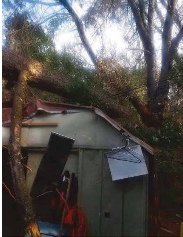
Figure 1: In Oroville, Butte County, a fallen tree hit a shed and eable wire service line . The tree also came into contact with the service drop (not shown).
