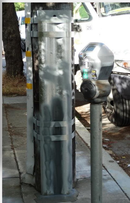
Finished job with steel truss banded to the pole.
