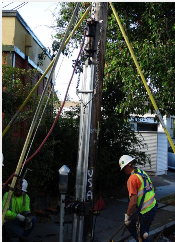
Typical Pole Reinforcement job showing crew ready to drive steel along side of pole. Work typically takes one hour at the location from start to finish.
