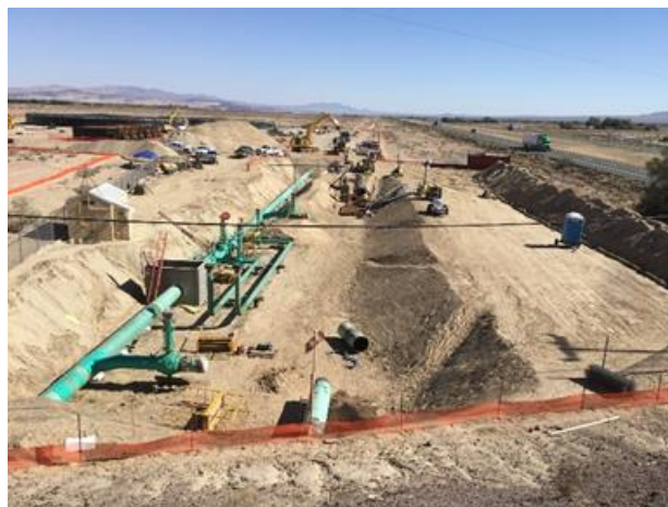
Figure 37 – Strength Test in Progress
