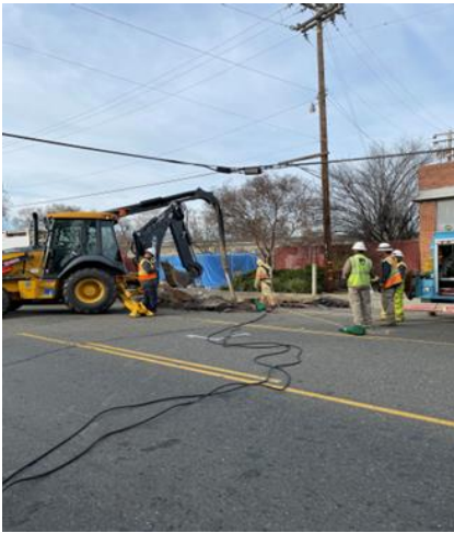
Figure 42 – PG&E’s Maintenance & Construction Crew at Work
