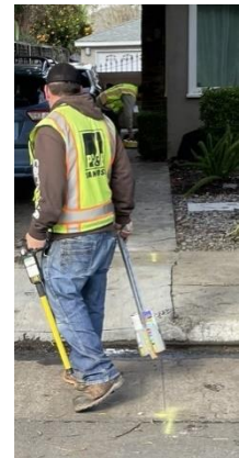
Figure 28 – PG&E Coworker Marking a Gas Main and Service
