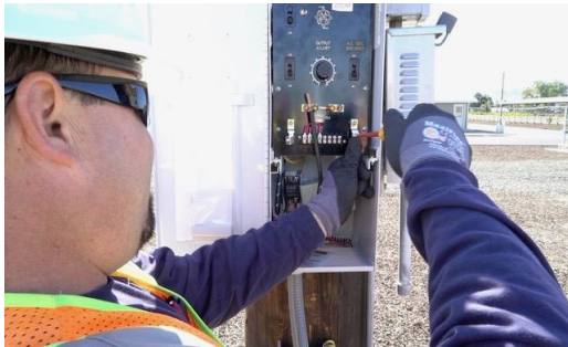
Figure 40 – PG&E Employee Installing a Cathodic Protection Rectifier
