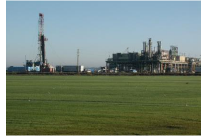
Figure 17 – Rig and Well Platform
