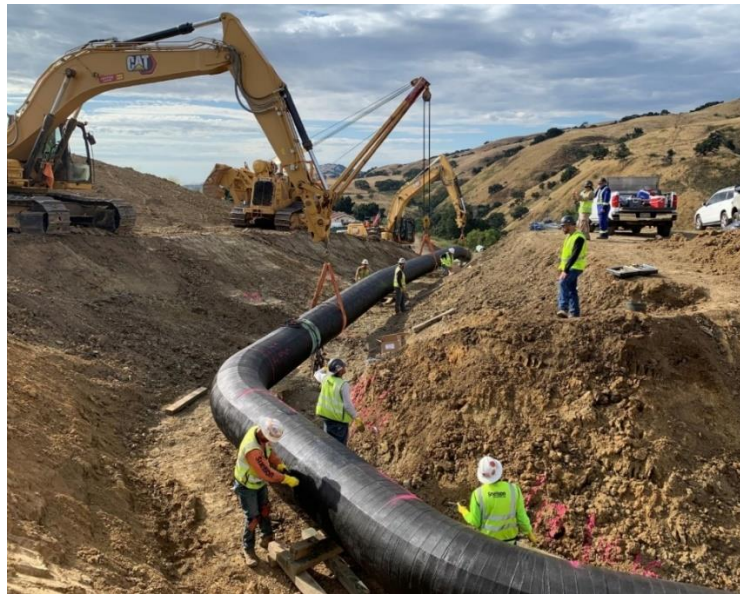
Figure 68 – Field installation of the advanced distributed fiber optic sensor monitoring systems on L-300B at a Calaveras Fault-crossing site in Gilroy.
