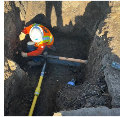
Figure 22 – Employee Working on Distribution Main and Service
