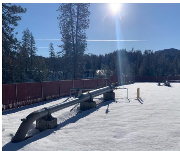
Figure 19 – Line 177A Launcher at Harrison Gulch
