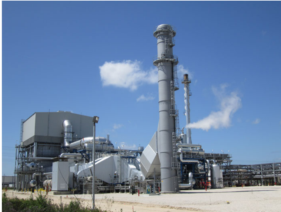
Steam reforming unit open in 2012 by Air Liquide in La Porte (TX)
