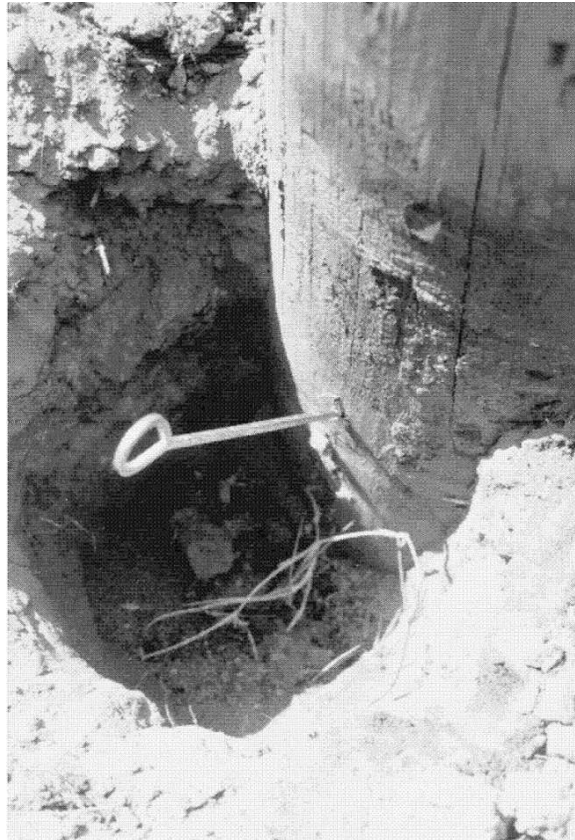
Figure 3. Using a Shell Thickness Gauge
