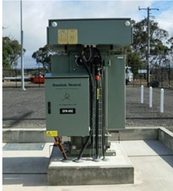
FIGURE PG&E-7.3.3-5: ARC SUPPRESSION COIL / GFN
