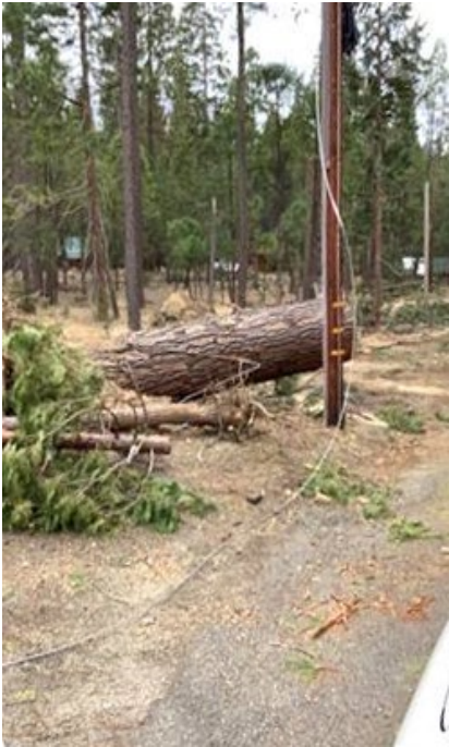
Figure 20: Vegetation-Caused Damage in Mariposa County – Tree Fell Through Line Breaking Conductor & Crossarm
