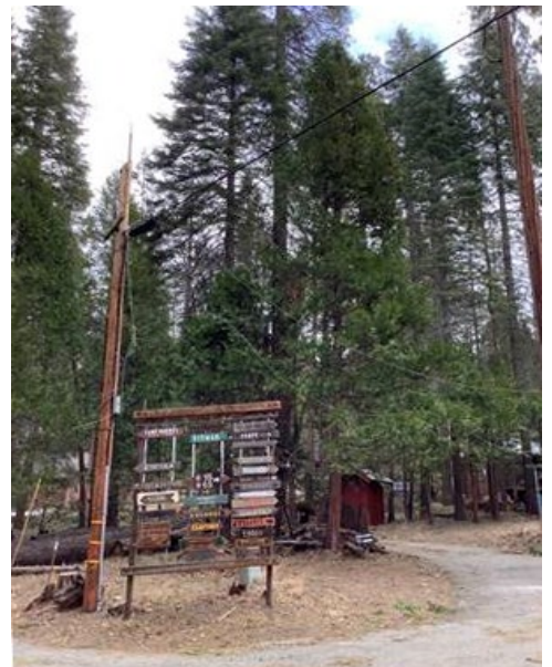
Figure 19: Vegetation-Caused Damage in Mariposa County – Fallen Tree Broke Top Half of Pole Off
