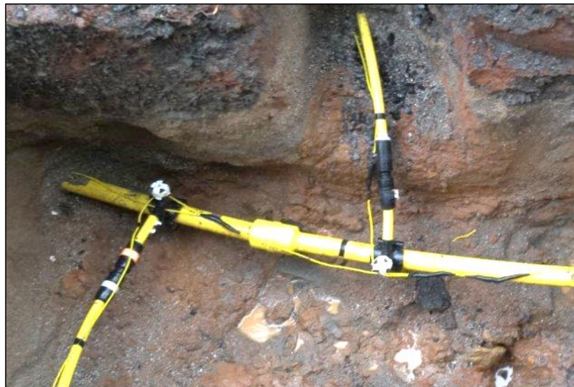
Figure 1. Daylighting a Facility
