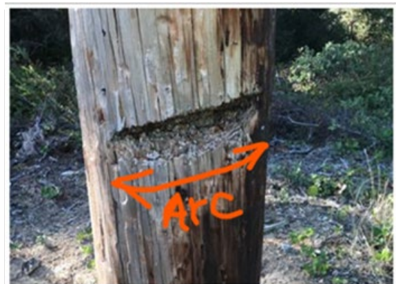
Figure 2: Definition of Crosscut Arc Length
