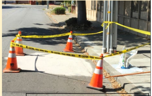
AFTER - Taped off, cleaning measures applied, stand by still
