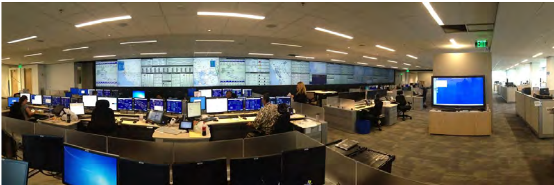
Figure 40 – PG&E’s Gas Control Center Features a 90 Foot-Long Video Wall With Current Operational Information to Augment The Gas SCADA System (Photo Captured Pre COVID-19)
