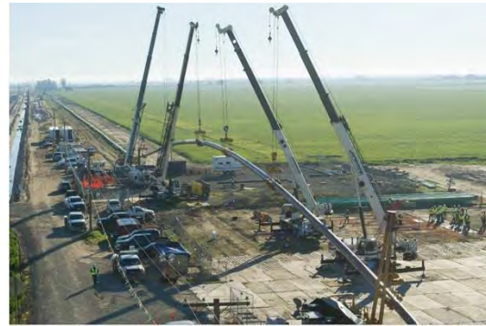
Figure 14 – Line 215-1 installing 24” pipe at Patterson
