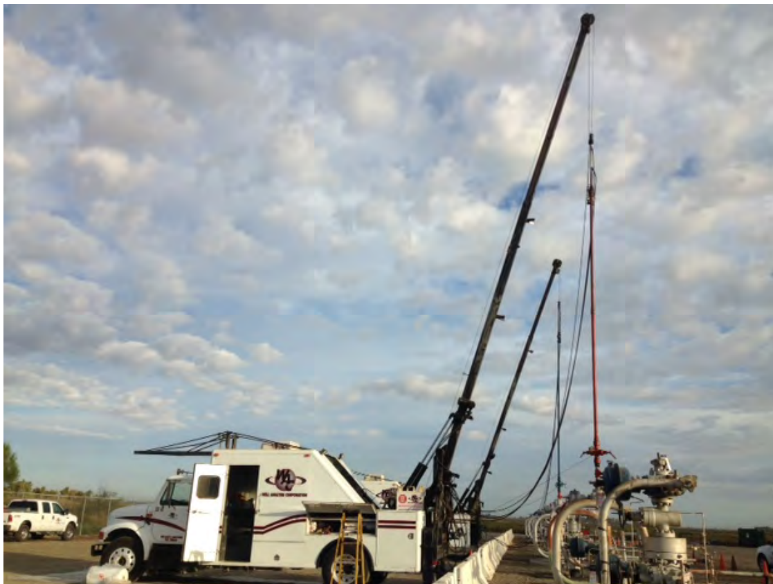
Figure 4. Temp/noise survey in progress on the Whiskey Slough station.
