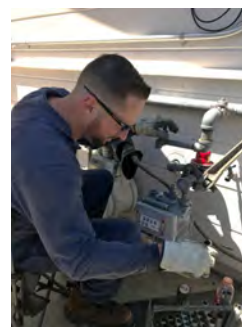
Figure 18 – PG&E Employee Working on Customer Connected Equipment (Photo Captured Pre COVID-19)
