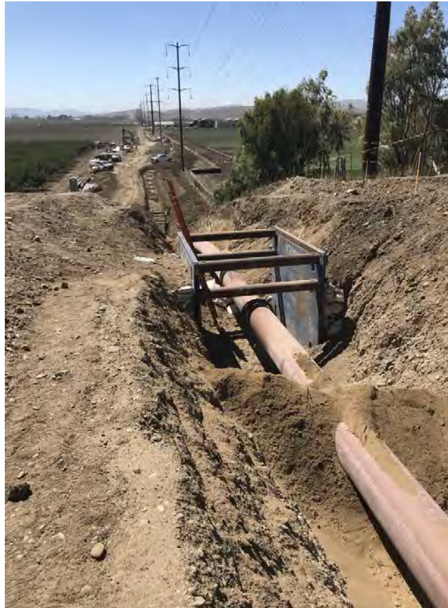
Figure 34 - L-301A Fault Crossing Pipe Replacement
