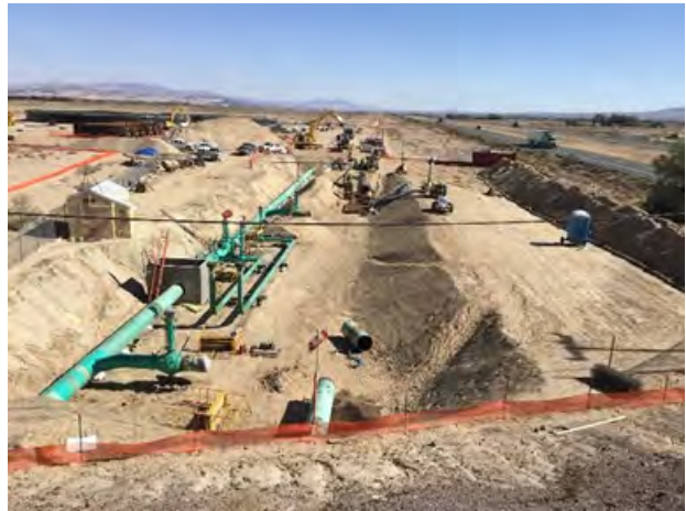
Figure 29 – Strength Test in Progress
