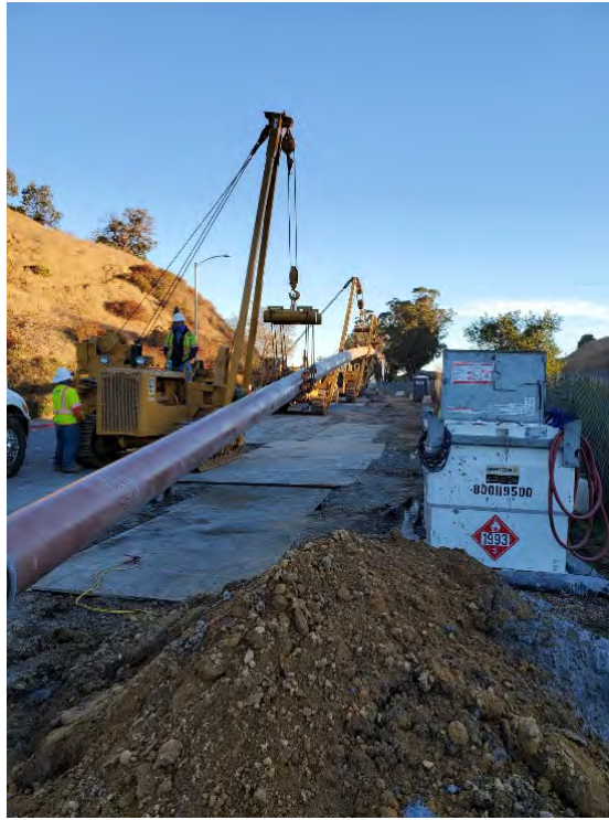
Figure 30 – Vintage Pipe Replaced in San Rafael
