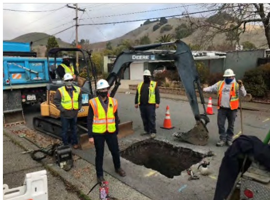
Figure 35 – PG&E’s Maintenance & Construction Crew at Work
