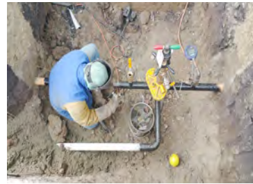
Figure 17 – Employee Working on Distribution Service
