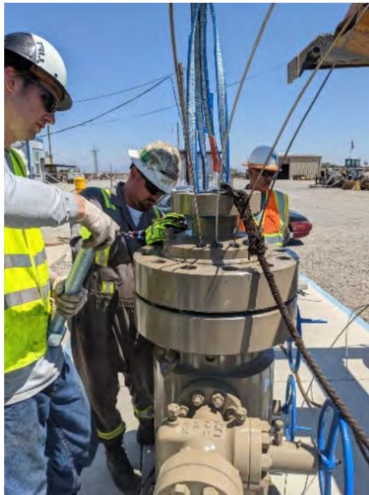
Figure 62 - Installation of Optical Fiber Sensors in a storage well
