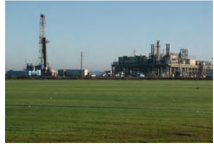
Figure 12 – Rig and Well Platform
