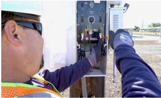
Figure 33 – PG&E Employee Installing a Cathodic Protection Rectifier (Photo Captured Pre COVID-19)
